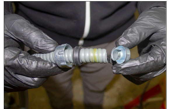
Figure 4-7: Flex conduit fitting assembly.
