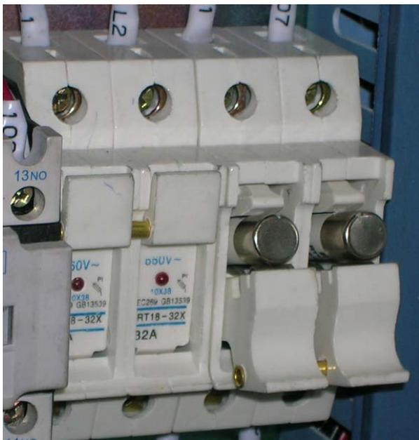
Figure 2 - Fuse block opened
