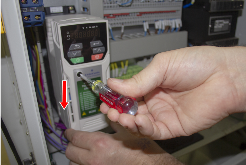
Figure 12: Removing the cover from the VFD.
