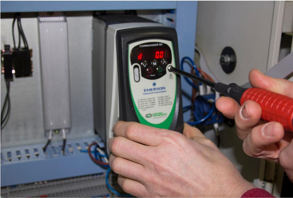
*Figure 19: Removing the faceplate from the VFD.*
