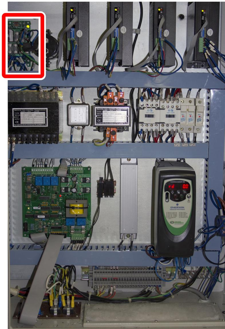
*Figure 24: DC-BUS board in the electrical cabinet.*
