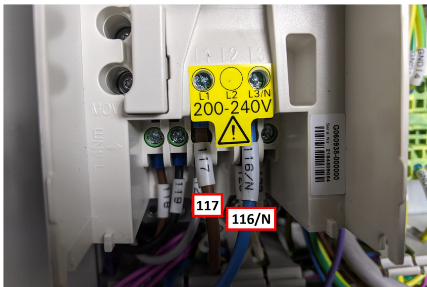
Figure 32: VFD wiring.
