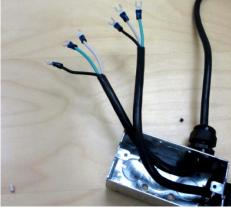
Both white wires will go to the terminal with the silver colored screw marked as terminal N.
