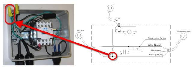
Grounds are all connected to each other with a wire nut. The grounds are the green wires.
