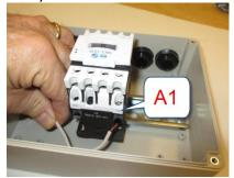
The cut ends of the extension cord are then run through the cord grips and stripped. The black wires of each should be stripped about 3/8" and the green and white wires are stripped about 3/4". The black wires will go to the contactor on terminals LI and T1. All this is summarized on the next page in both photo and schematic.
