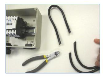
Next cut the 10' extension cord approximately in half. Also cut off a short section of about 12" as we'll need a bit of wire for the internal wiring. Pull each of the individual wires out of the short bit of cord.
