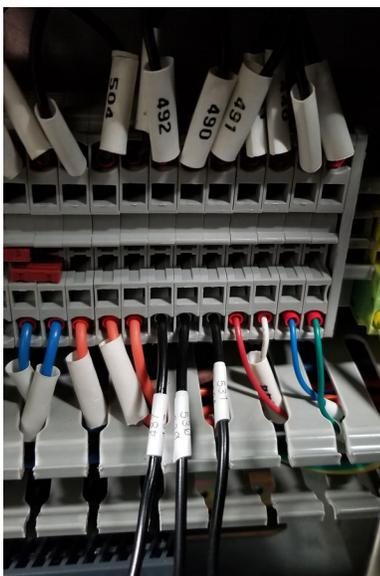
Figure 35: Wires 530 and 531 connected to the terminal block.
