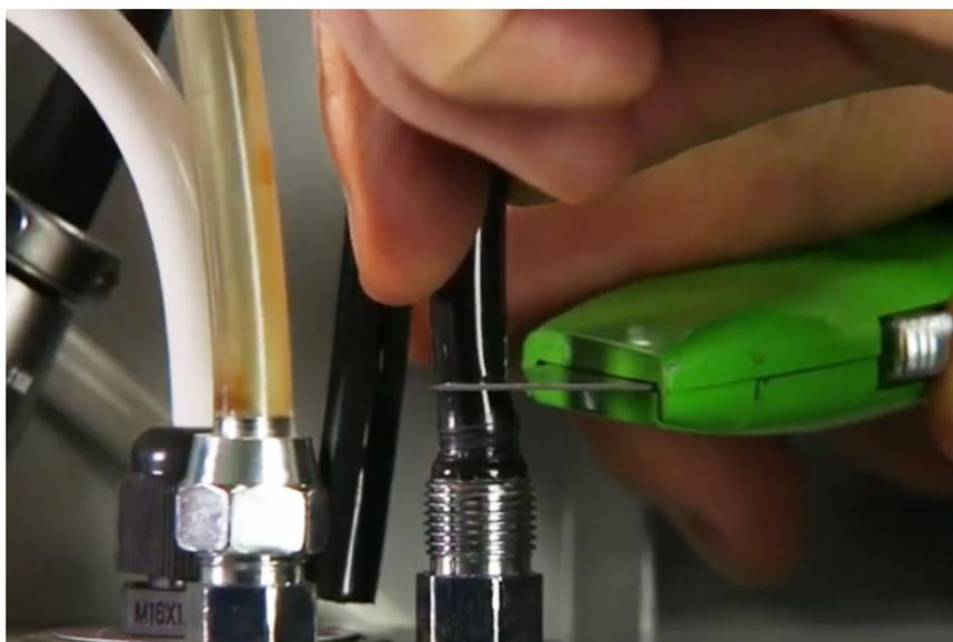
*Figure 5: Cutting the water lines from the fitting.*
