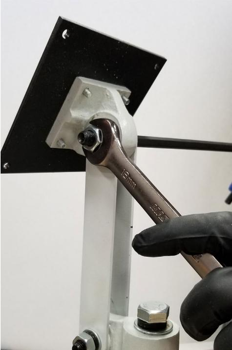
*Figure 4: Tightening the monitor bracket in place.*
