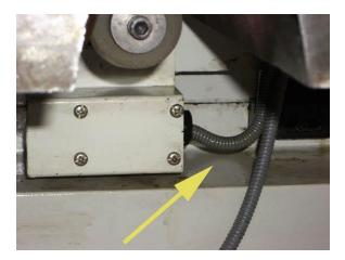
Figure 3 - Cable with drip leg
