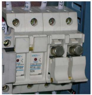
Figure 2 - Fuse block opened
