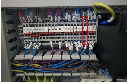
Figure 5: Empty terminal block moved next to 102 N terminal blocks.
