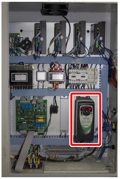
Figure 18: VFD in the electrical cabinet.
