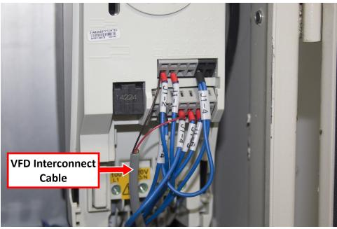
Figure 20: VFD interconnect cable connected to the VFD.
