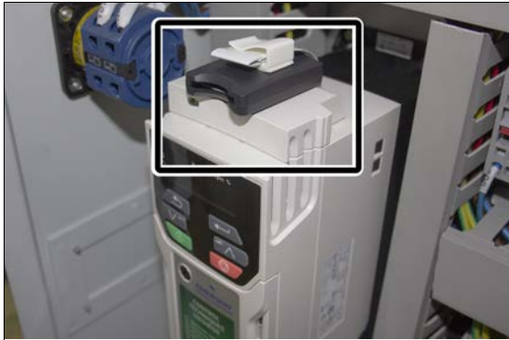
Figure 2-1: SD Card Programming Adapter installed on the VFD.
