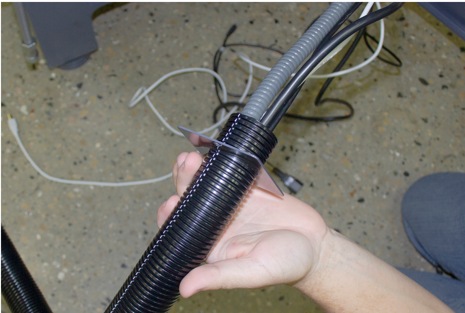
Figure 21: Loose end of corrugated tubing and all cords put through the access panel.
