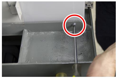
Figure 14: Securing the left side panel to the machine stand.
