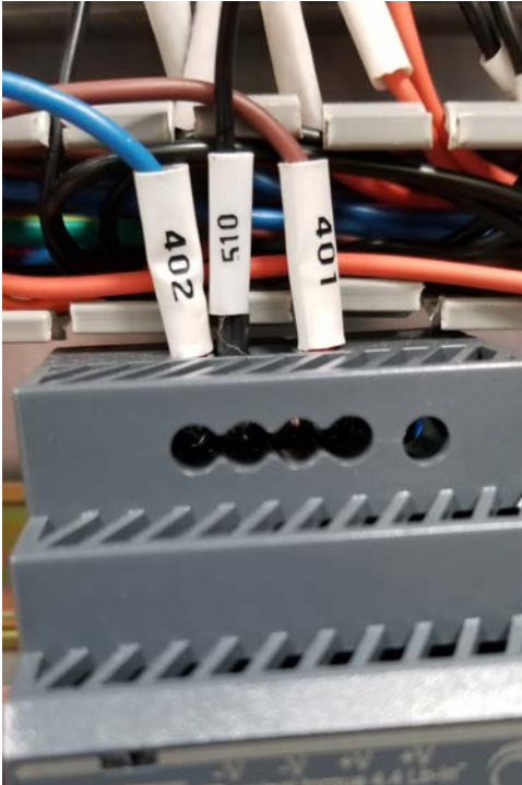
Figure 7: Wire 510 on the V- terminal on the power supply.
