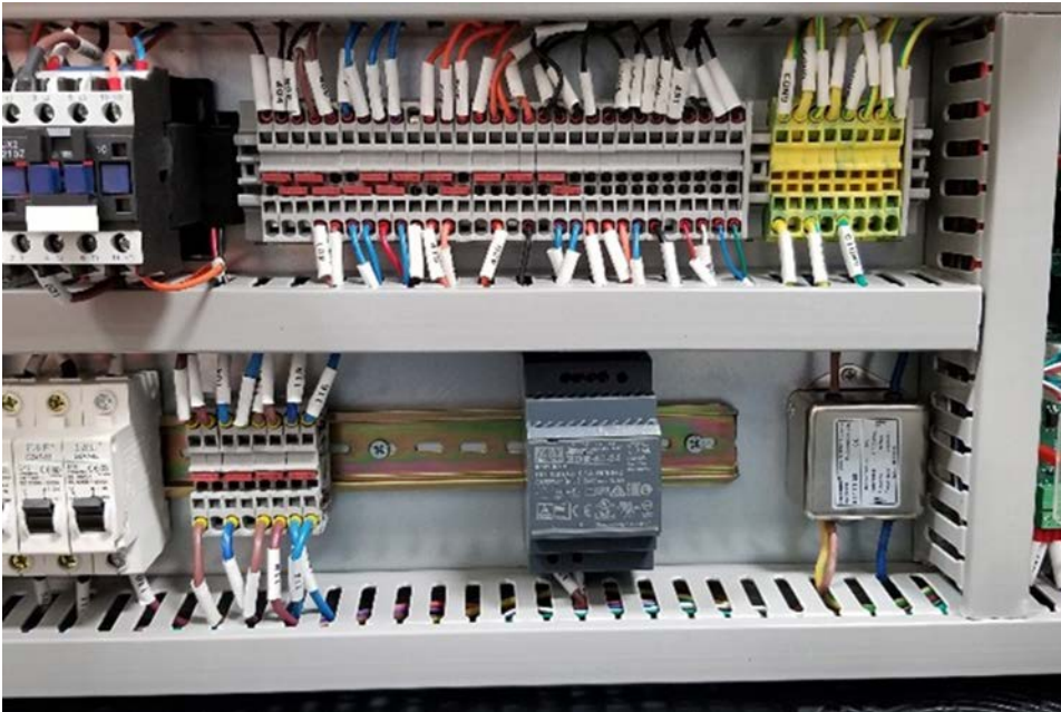
Figure 7: Wire troughs re-installed.
