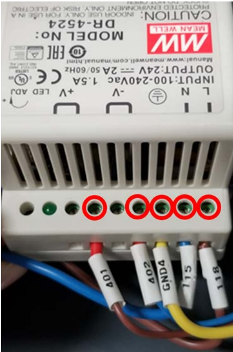
Figure 3: Wires to remove from the existing power supply.
