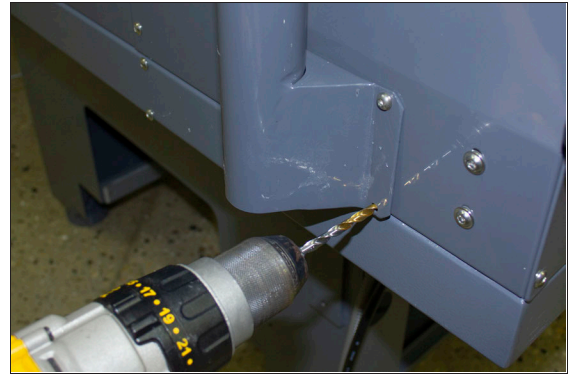
Figure 4-178: Drilling the remaining three holes into the enclosure.
