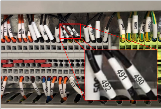
Figure 4-57: Wires 490, 491, and 492 connected.
