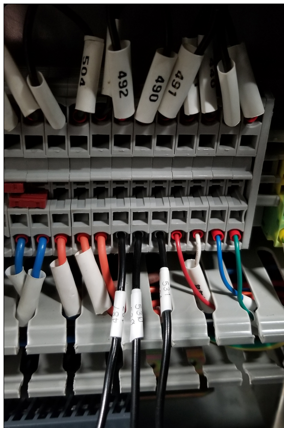
Figure 4-78: Wires 530 and 531 connected to the terminal block.
