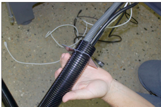
Figure 4-161: Loose end of corrugated tubing and all cords put through the access panel.
