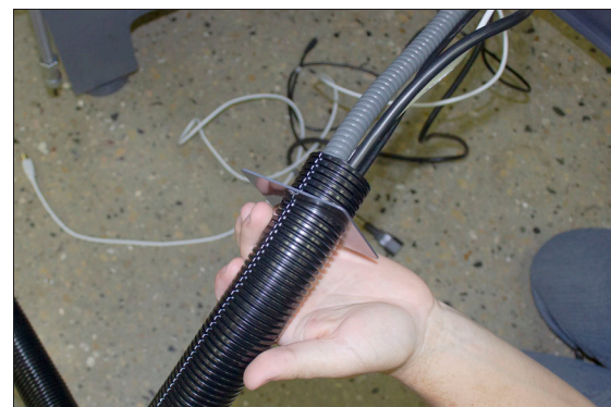
Figure 4-154: Loose end of corrugated tubing and all cords put through the access panel.
