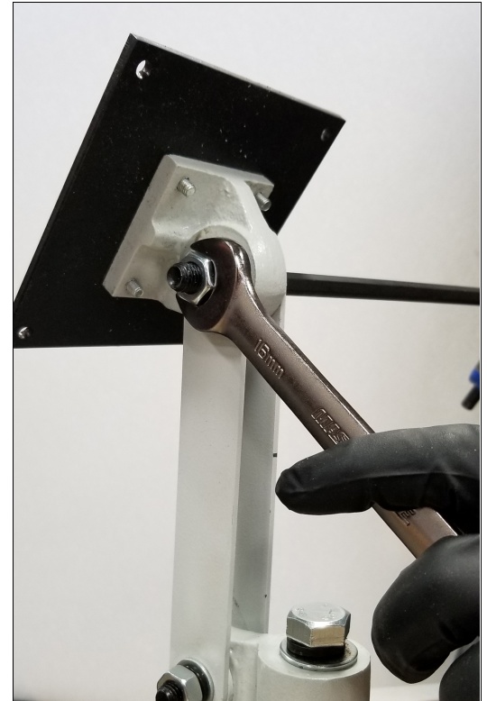
Figure 4-10: Tightening the monitor bracket in place.
